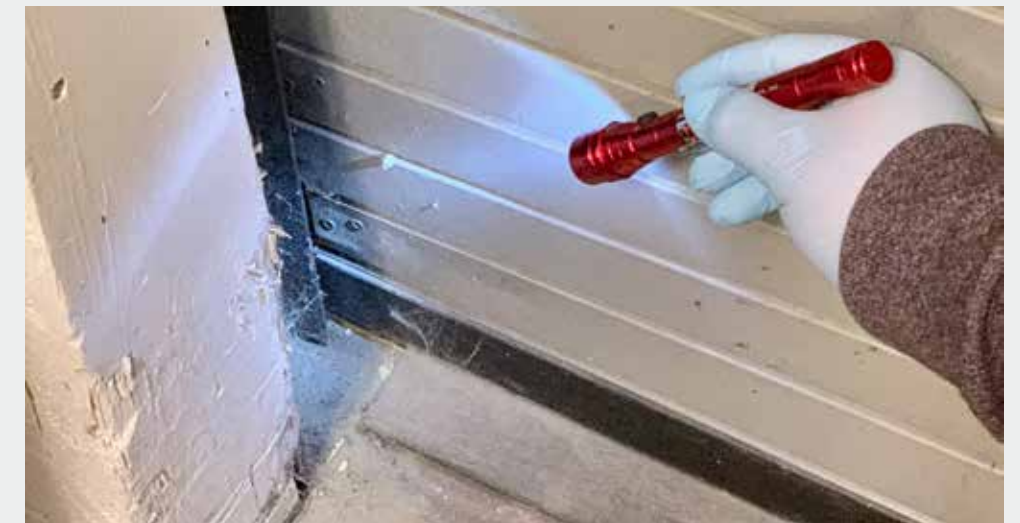
Inspecting loading docks for evidence of rodents
