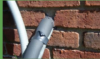
Around HVAC Lines
